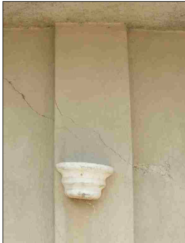
Figures 3.63 and 3.64 Shear cracking on side faces: earthquake damage (Sedra, et al. 2010)
