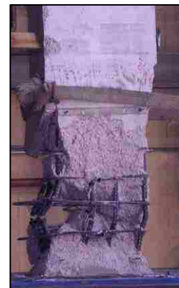
Figure 3.21 (F8) Longitudinal Bar Fracture
