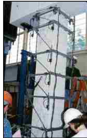
Figure 3.23 (S1 & S2) Flexural and Shear Cracking
